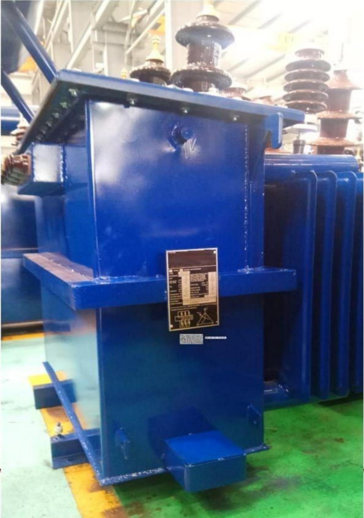
**TECHNICAL SPECIFICATION OF 100 KVA, 11/ 0.433 KV and 22/ 0.433 KV, Star 1 (Level-1) THREE PHASE, OIL IMMERSED, OUTDOOR, NON SEALEDTYPE DISTRIBUTION TRANSFORMERS WITHOUT CSP FEATURE**
